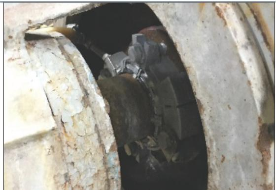
442C Cartridge Split Seal 114 mm (4.50") was installed in less than two hours.
